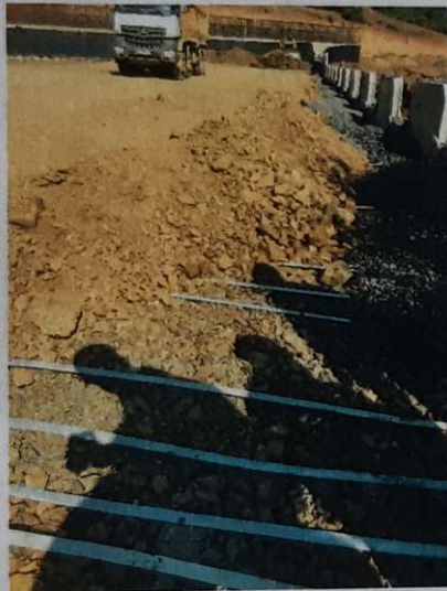
Figure 4&5: Strips and panels are used to reinforce earth.
