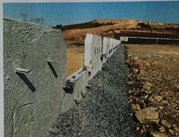
Figure 4&5: Strips and panels are used to reinforce earth.
